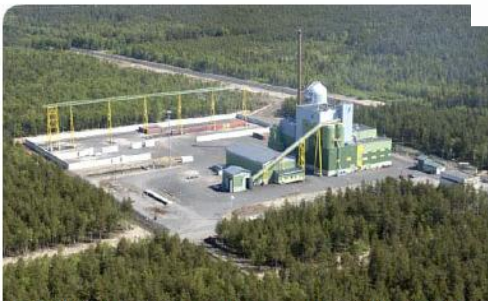
The 20 MWe Kokkolan Voima power plant was completed in 2001 and is fired on a mix of wood, field energy crops, and peat. Copyright Pohjolan Voima Oy
